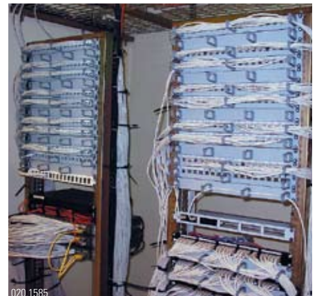
Flexibility: Patch panels each with 16 connections.
