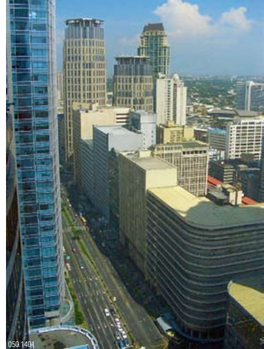
050 1401 View from Henkel office located in the busy business district in Makati
