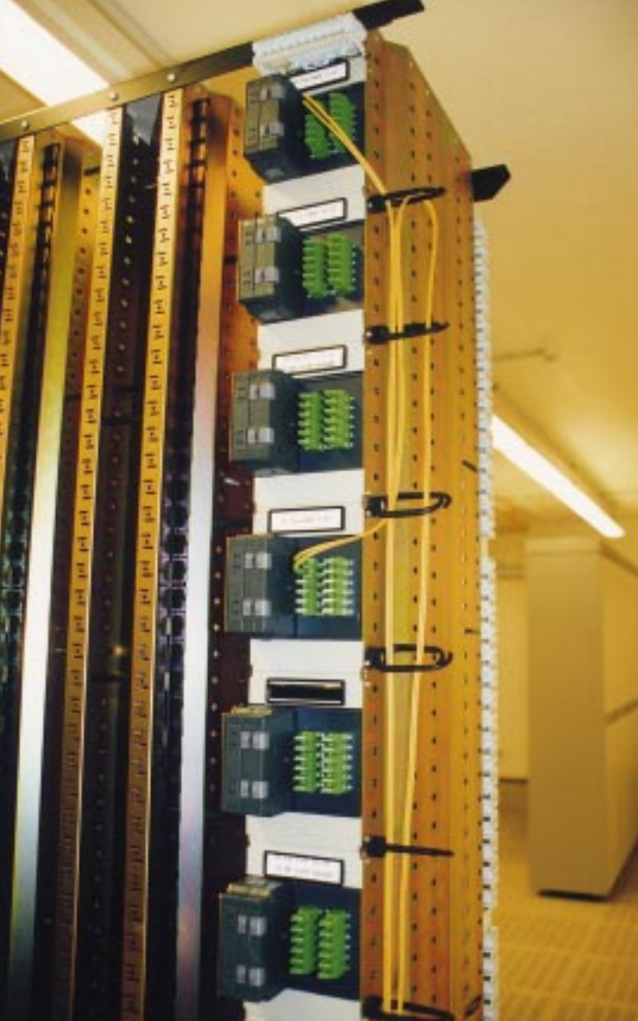
FO mounting channel solution CT
