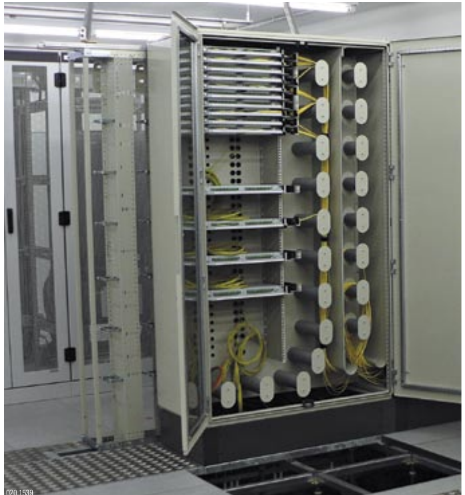
R&M FOM distributor with Uniracks including drag chain guide and double overlength management.
