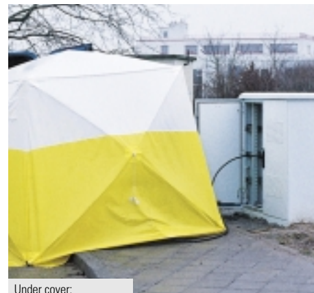
Under cover: Installing cables in the distribution cabinet.
