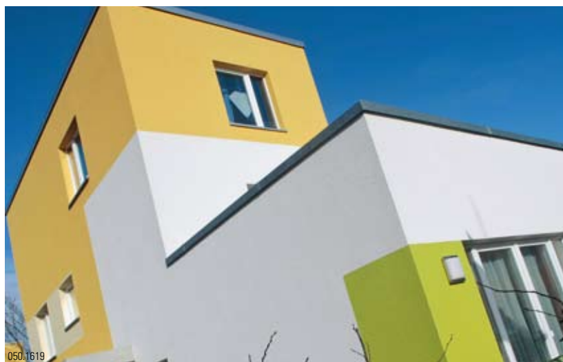
Within a few months 130 000 apartments were catapulted into the ultra broadband era.
